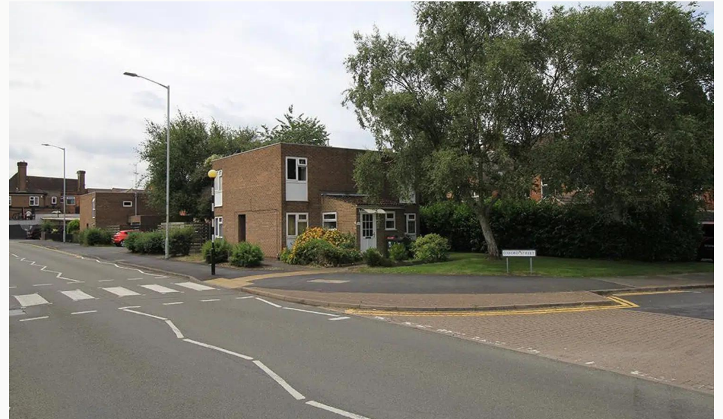
Front of Building
